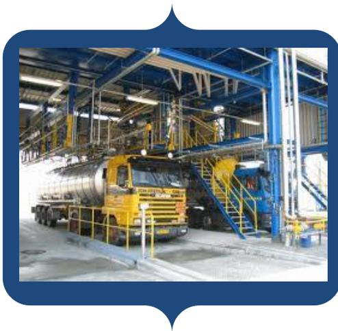
& the loading rack are operated manually by the on-site operator who will also aid the truck driver in any case. The correct line-up of the valves will be the operator's responsibility, if the valves are manual, else complete valve automation will be provided. The ESD valves will be shut down in case of any ESD condition. ESD may be system invoked or manually invoked from the ESD buttons. ESD will need to be reset from the HMI.
